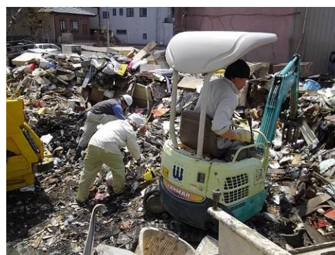
Members in Hyogo Prefecture helping clean up the community in Miyagi
